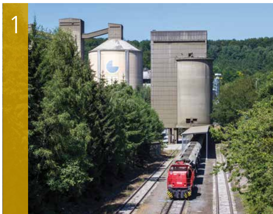
1. IMPIANTO DI CARICO DEL CLINKER A RUMELANGE (FOTO: JÖRG KLAWITTER) CLINKER LOADING SYSTEM AT RUMELANGE (PHOTO: JÖRG KLAWITTER)
